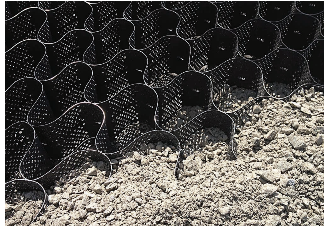
Figure 9. Geocells partly filled with aggregate
