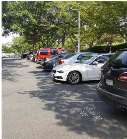
Before: asphalt pavement
