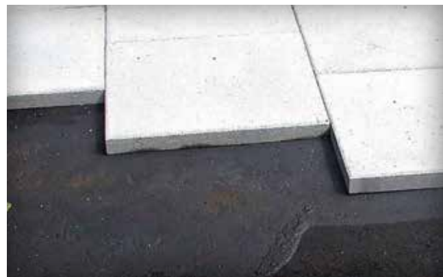
Figure 8. Sidewalk application illustrating the neoprene adhesive on an asphalt bedding layer under paving slabs
