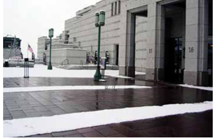
Figure 7. To conserve energy, the snow melt system is only installed directly under the high traffic areas where it is needed.
