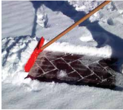
Figure 4. Shovel snow diagonal to the paver pattern to prevent catching edges.
