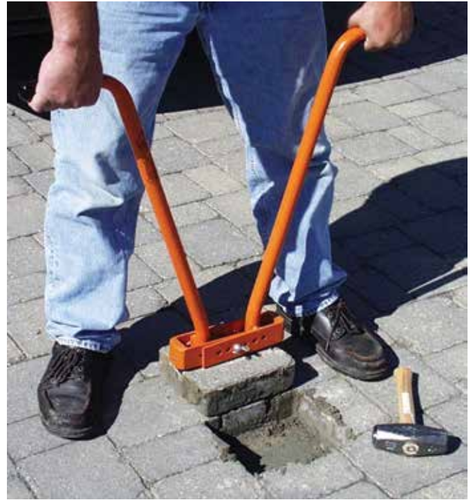
Figure 30. A paver extractor can be used to grab the first paver and wiggle it out.
