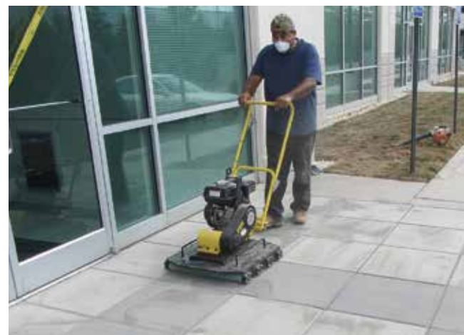
Figure 19. Compacting paving slabs with a roller attachment on a plate compactor
