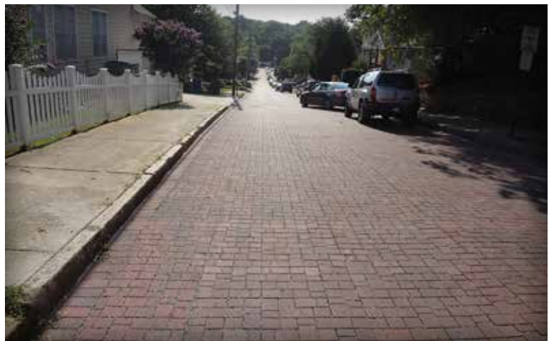
Figure 1. PICP is seeing increased use in municipal streets to reduce stormwater runoff, local flooding, storm pipe upsizing, and combined sewer overflows. These streets are in Atlanta, GA.
