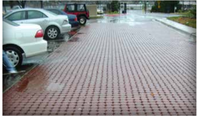
Figure 11. Ponding on PICP typically first occurs at the junction with impermeable pavement.
