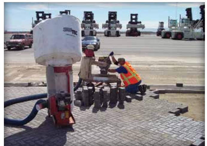
Figure 8. Saw cutting pavers.
