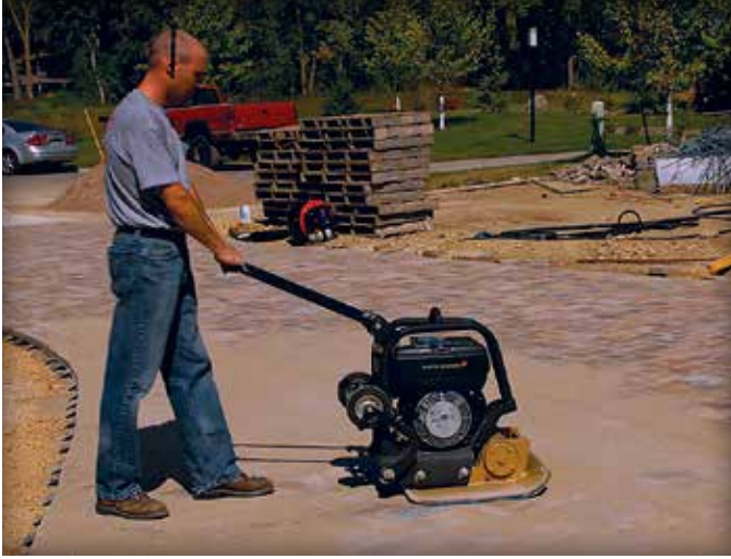
Figure 11. Vibrating sand into the joints.
