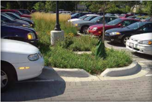
Figure 5. Elmhurst College, Elmhurst, Illinois parking lots uses full infiltration through the soil subgrade with overflows directed through curb inlets into bioretention areas and overflow drains to manage extreme rain events.
