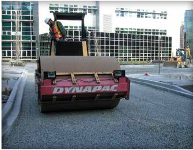
Figure 20. A 10 ton (9 T) roller compacts the ASTM No. 57 base.
