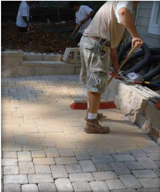
Figure 8. Spreading joint sand over the installed concrete pavers.
