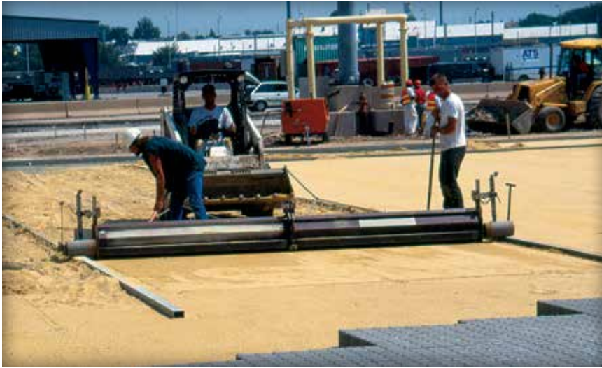
Figure 17. Powered screed bucket accelerates spreading of bedding sand. The width of the bucket can be adjusted.
