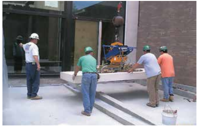
Figure 13. Large vacuum head lifts an oversize paving slab
