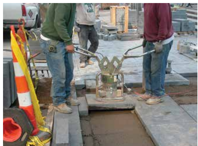
Figure 15. Two-person vacuum lift for larger paving slabs.
