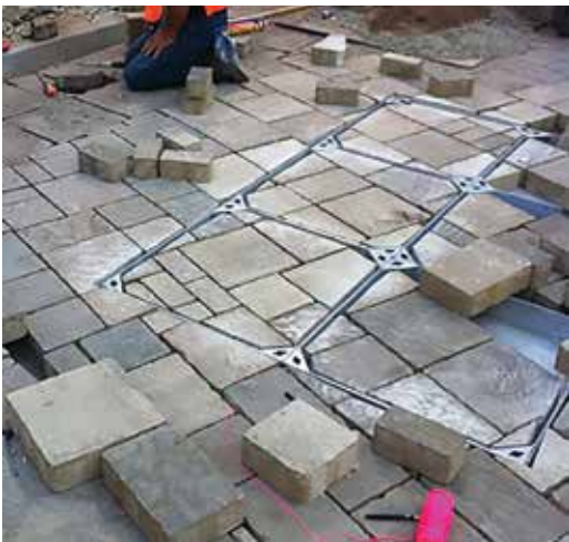
Figure 28. Another example of cutting pavers to accommodate a utility cover set at an acute angle to the paving slab pattern
