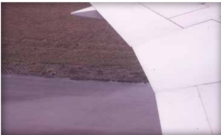
Figure 11. Airfield taxiway shoulder
