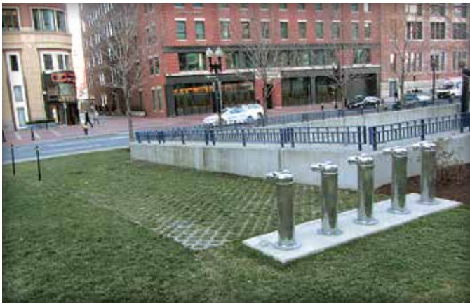
Figure 7. Emergency access lane for fire trucks
