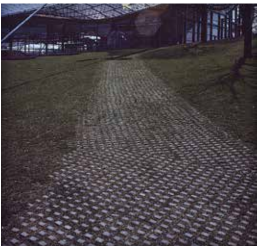
Figure 6. Service access lane
