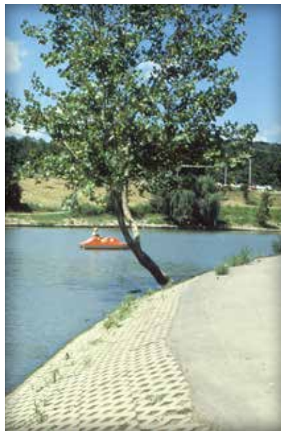
Figure 4. Lakeside stabilization
