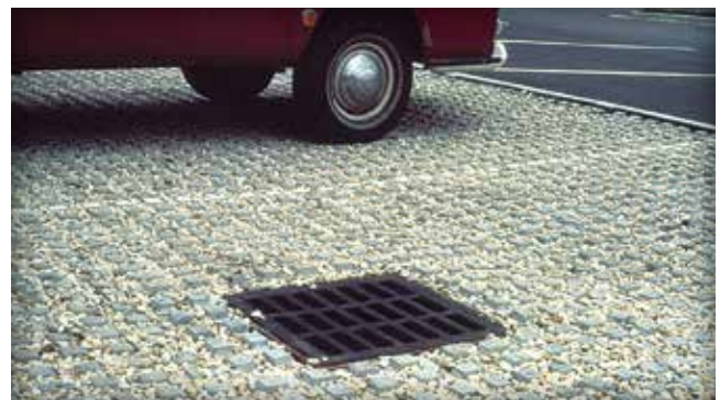
Figure 16. Concrete grids with aggregate in the openings
