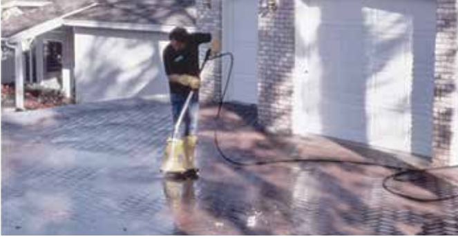
Figure 11. Pressure washers are commonly used to clean ICP. When using be careful not to remove joint sand.
