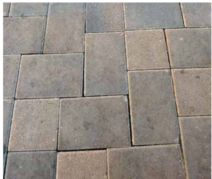
Figure 20. Variation in the joint width is a typical present in ICP with excessive joint width.
