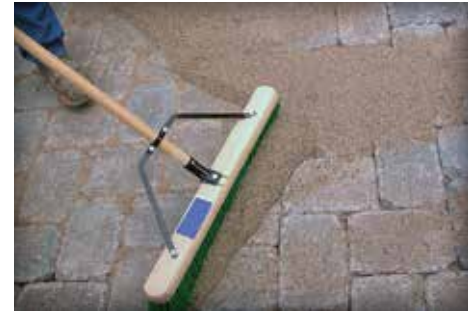
Figure 5. Joint sand can be pre-mixed and delivered to the site (typically in bags), or mixed with stabilizer at the site, then swept into the joints, compacted for consolidation in them to create interlock, and wetted to activate the stabilizer.
