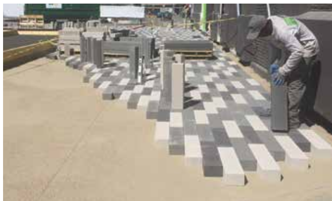
Figure 6. Installing planks on uncompacted bedding sand.
