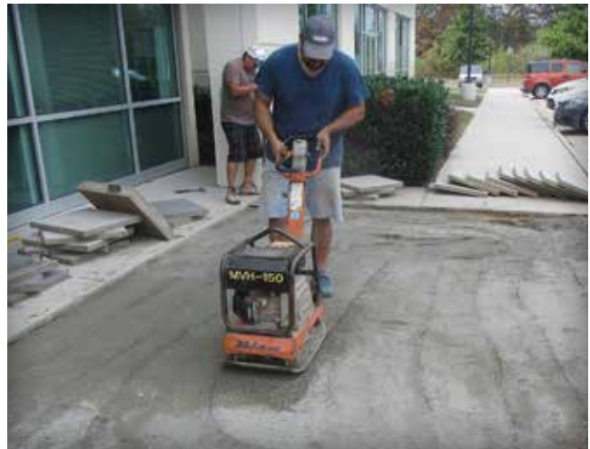
Figure 5. Precompacting the bedding sand
