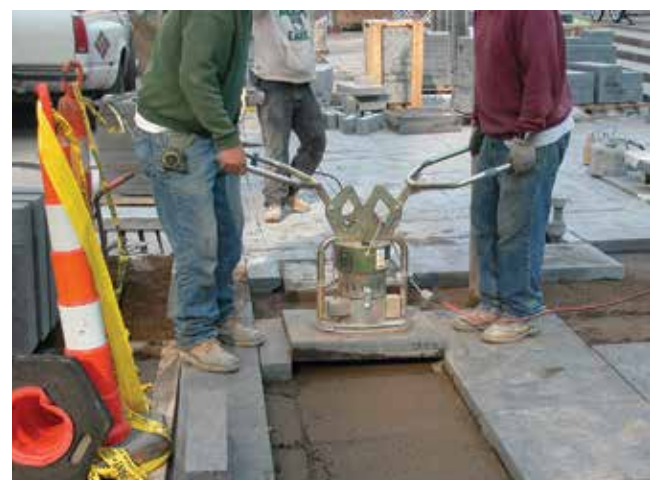
Figure 15. Two-person vacuum lift for larger paving slabs.
