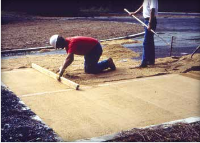
Figure 6a & 6b. Screeding the bedding sand.
