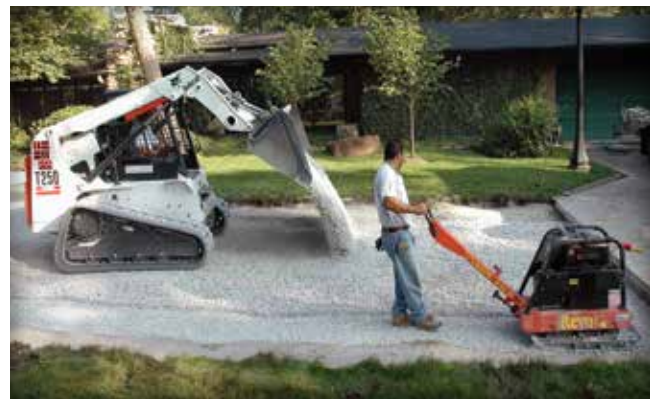
Figure 18. Compacting the berms along the perimeter and the PICP base
