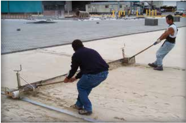
Figure 4. A two-man hand pulled screed
