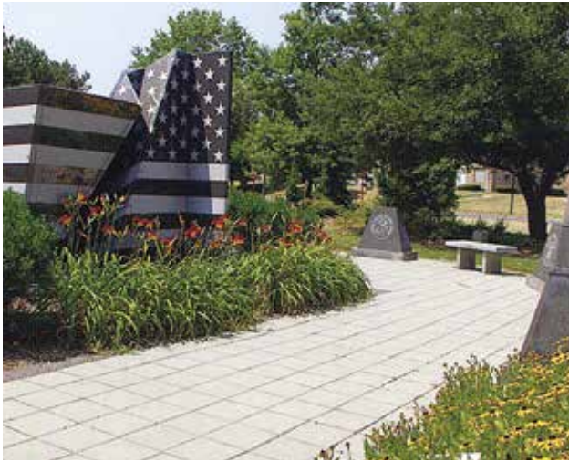
Figure 14. High SR paving slabs
